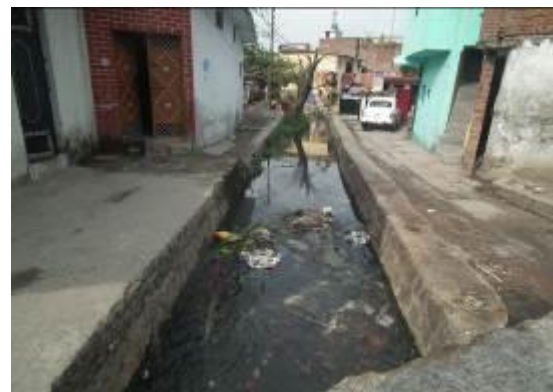
Raw sewage is flowing in natural water drains (Existing conditions)
