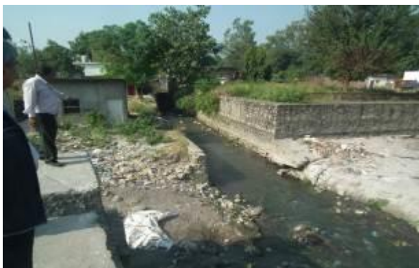
Raw sewage is flowing in natural water drains (Existing conditions)
